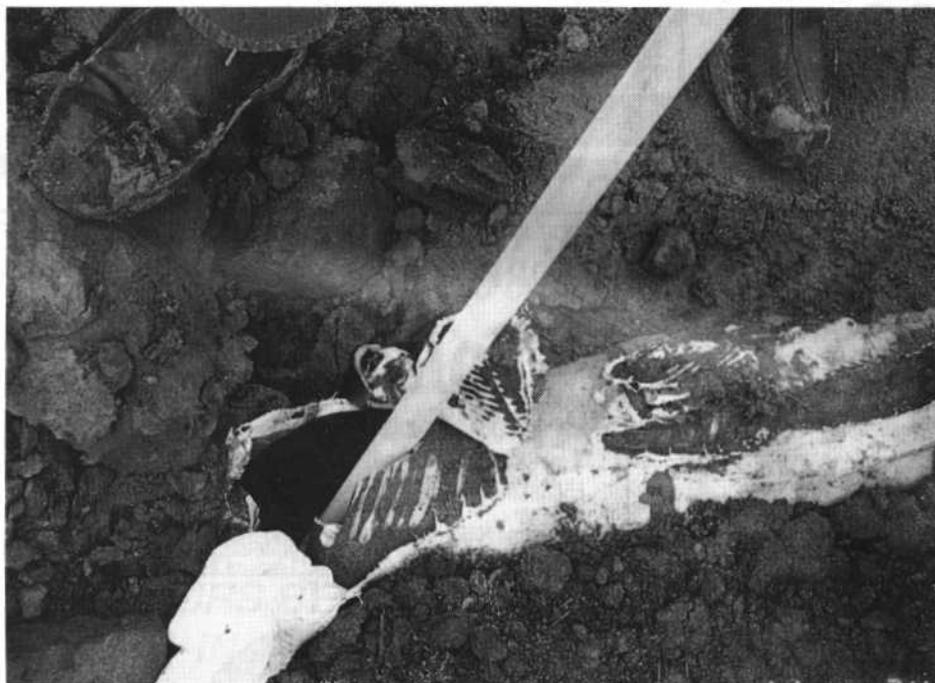
The blade of the scraper skimmed the top of the pipeline, while a guide tooth at the end of the blade went slightly deeper and gouged a hole in the line. The white rod is the end of a vacuum tool being used to clear the line prior to repair.
